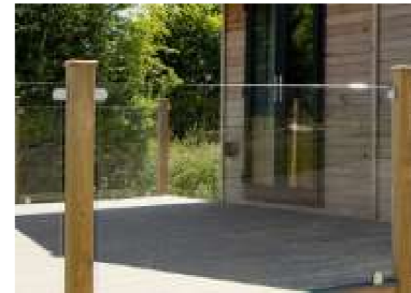
Glass in Stainless Steel Brackets between Timber Posts
