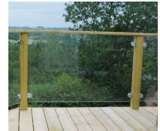
Glass in Stainless Steel Brackets between Timber Posts
