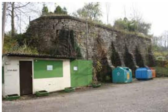
The kilns were built with large revetment walls, circa 1806, of coursed and roughly dressed sandstone, with ashlar blocks to the coping, archivolt and buttresses. The retaining wall is approx. 20m long and 7m high, and is buttressed by 6 inclined sections on the principal west elevation and with a short return to the north. The west elevation has two semi-circular arched stoke holes, set between pairs of inclined sections.
