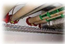
Contractors installing cables, pipes in buildings are obliged to fire stop cable holes through which they have cabled as part of the contract. All cable holes through floors and compartment walls must be fire stopped to prevent passage of fire, smoke and hot gases.
